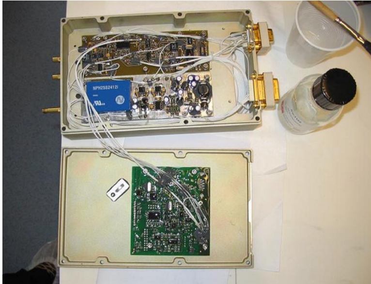
The S Band Control deck with PSU and the control board with the TNC on the lid The unit includes the 13cms exciter, the 3 watt PA from G3WDG, a switchmode power supply, a TNC, sensor board and control board.
